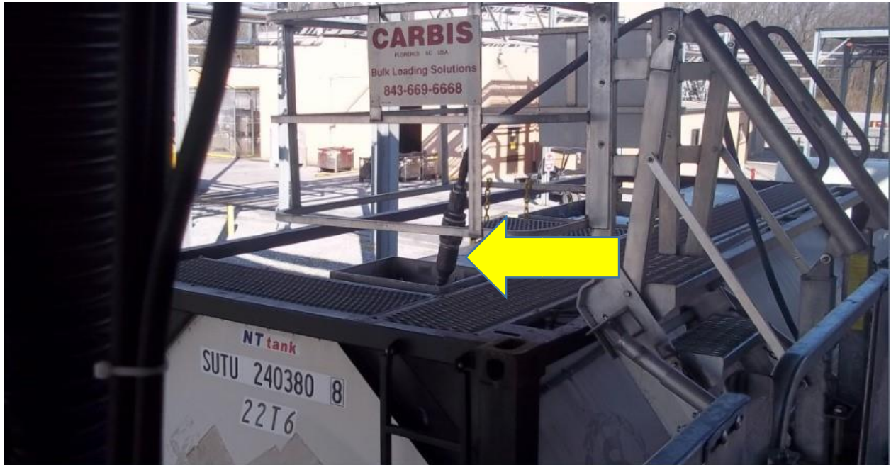
Acceptable vapor return or vent access
